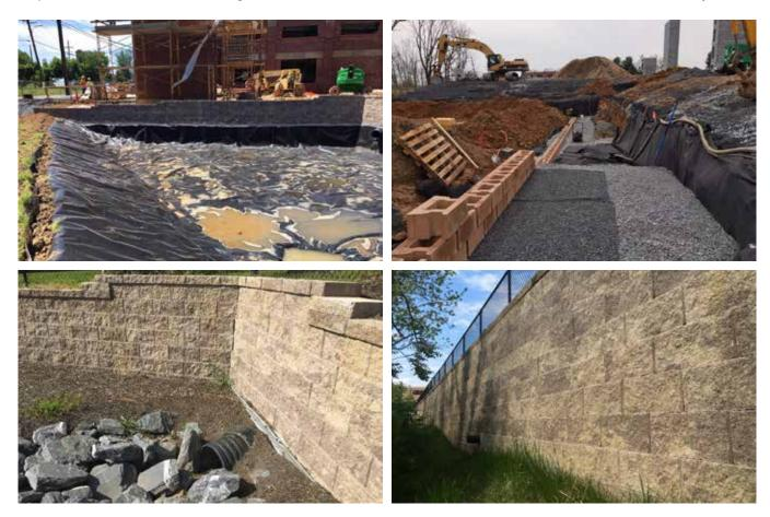
At its highest point of 13 courses tall, the retaining wall measured 8.67ft (2.64m), plus the cap unit. To withstand the rigorous weight and pressures of the vehicles and traffic, Strata SG200 geogrid was also chosen to reinforce the backfill for a stabilized base under the parking lot. This polyester geogrid material increases the retaining wall's strength. In turn, it significantly reduces the need for future repairs and maintenance.
